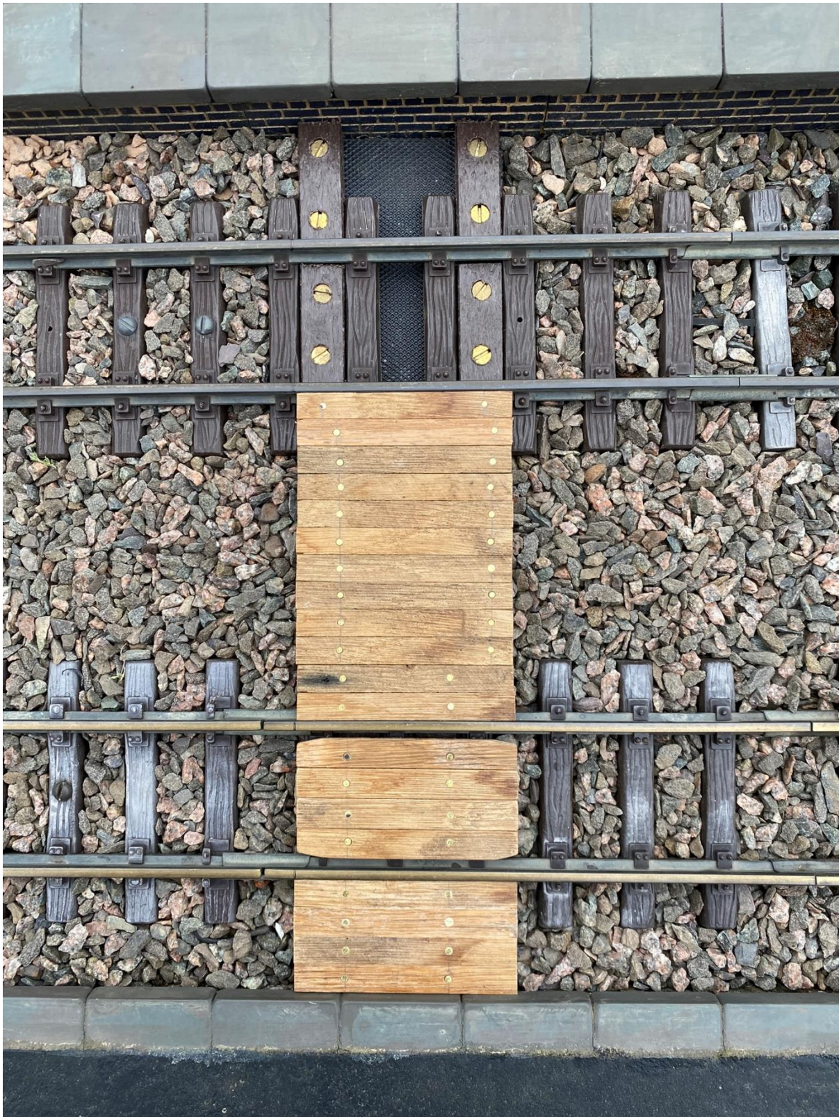
Picture 3: note the differing positions of the pins used to secure timbers to supports.
